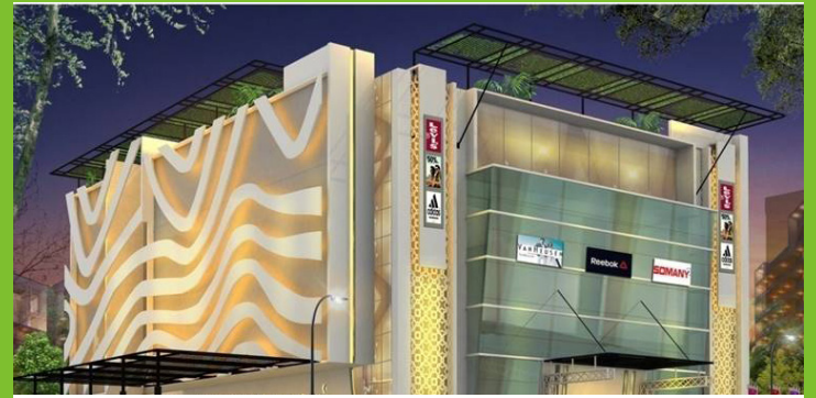
Commercial Building (NADAKKAVU)
